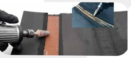
3. Solvent clean the buffed area with RS Rubber Buffer and apply RS-8400 rubber primer,
